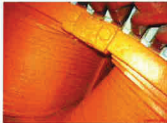
Figure 26: Humidity on the windings
