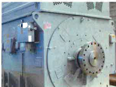
Figure 9: Machine with single bearing
