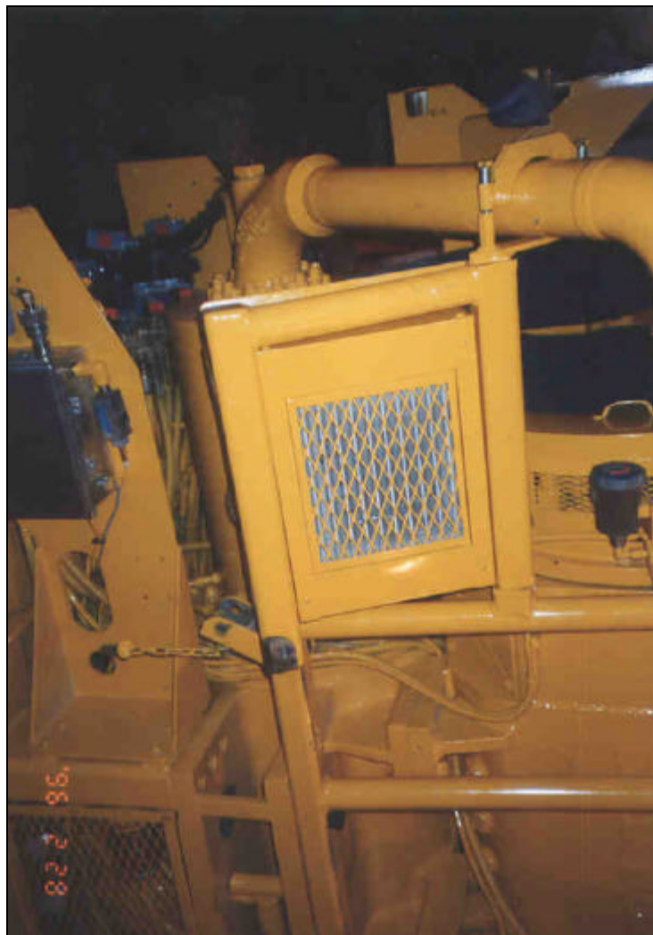
Figure 8-Insufficient Support
