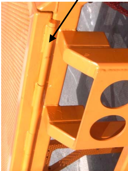
Figure 2. Upgraded Hinge detail
